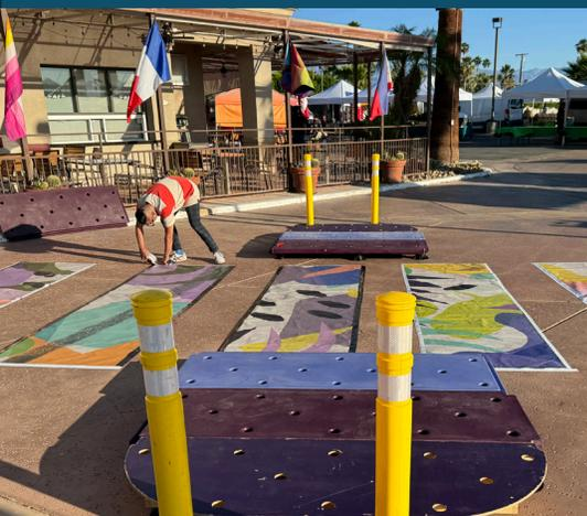
A median refuge island was installed to demonstrate how crossings can be optimized to decrease delays, reduce crossing distance, and minimize exposure to vehicular traffic.
